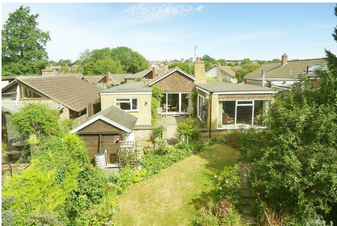
View of rear of house
